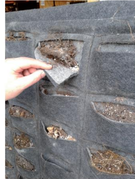
Fig. 6 Felt system may consist of different layers
